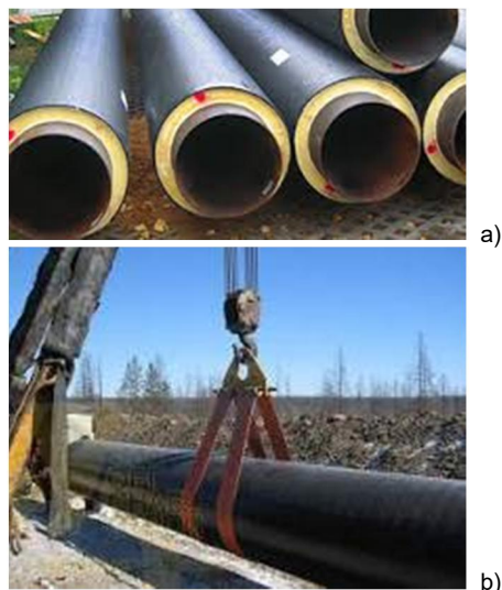
Figure 1 Components and way of laying oil and gas pipelines: a) pipes with external factory insulation coating; b) woven power grips
